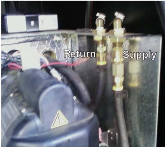
When you install the fuel lines make sure that you have connected the fuel supply and return lines in the correct places. Refer to photo above for burner connections and the one below to identify the lines.
